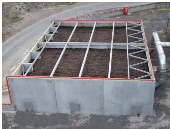
Extraction Plant Biofilter
