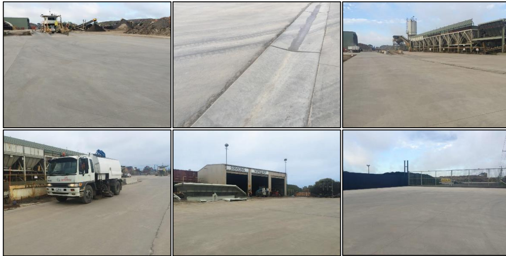
Figure 7 Site improvements at Sunshine Groupe
