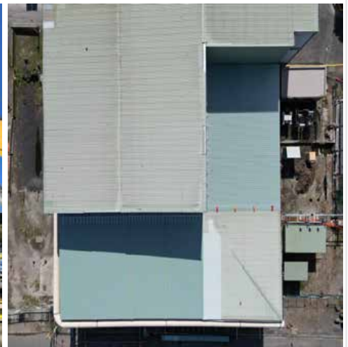
Roof replacement to be completed November 2022
