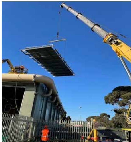
Roof replacement commenced July 2022
