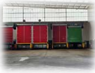
Rapid roller door replacement
